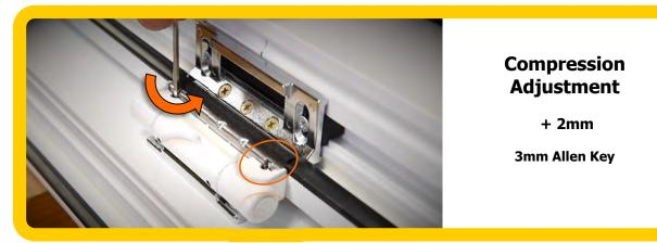
Open the Door to expose the Compression Adjustment Grub Screws Rotate the Grub Screws Anti-Clockwise to increase compression using a 3mm Allen Key Note both Grub Screws must be rotated by an equal amount to ensure even adjustment
